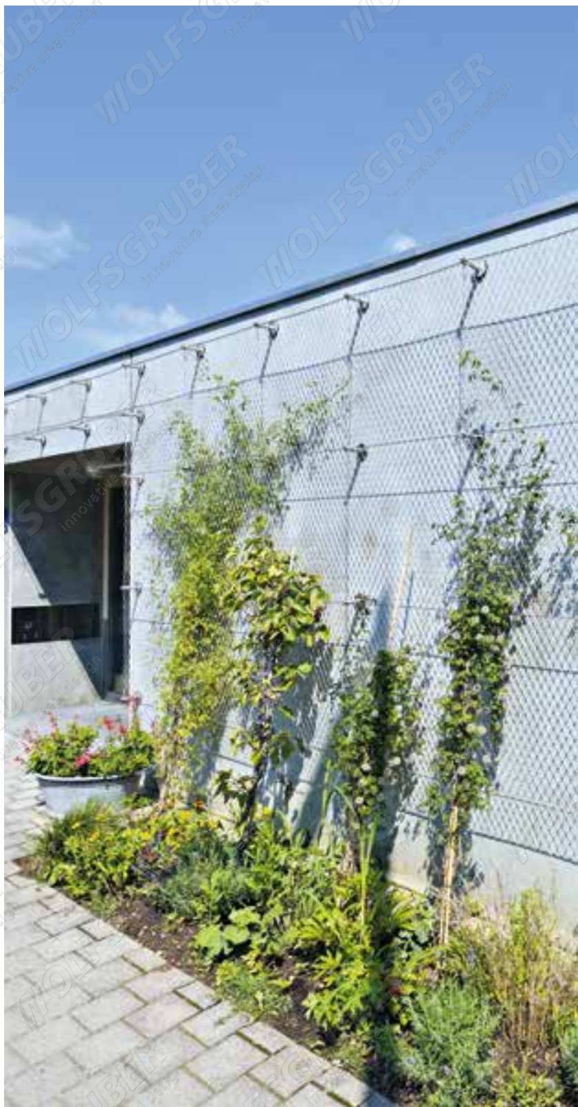
X-TEND CX / I-SYS 70 m 2 , \varnothing 40 mm, \varnothing 1,5 mm / \varnothing 4 mm
