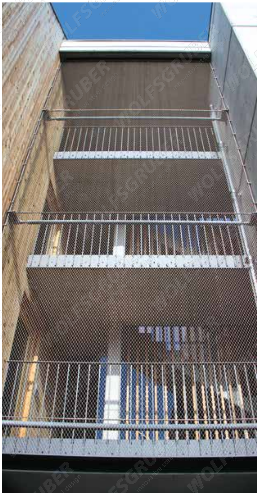
X-TEND CXE / I-SYS 120 m 2 , \diamond 30 mm, \circ 1,5 mm / \circ 12 mm
