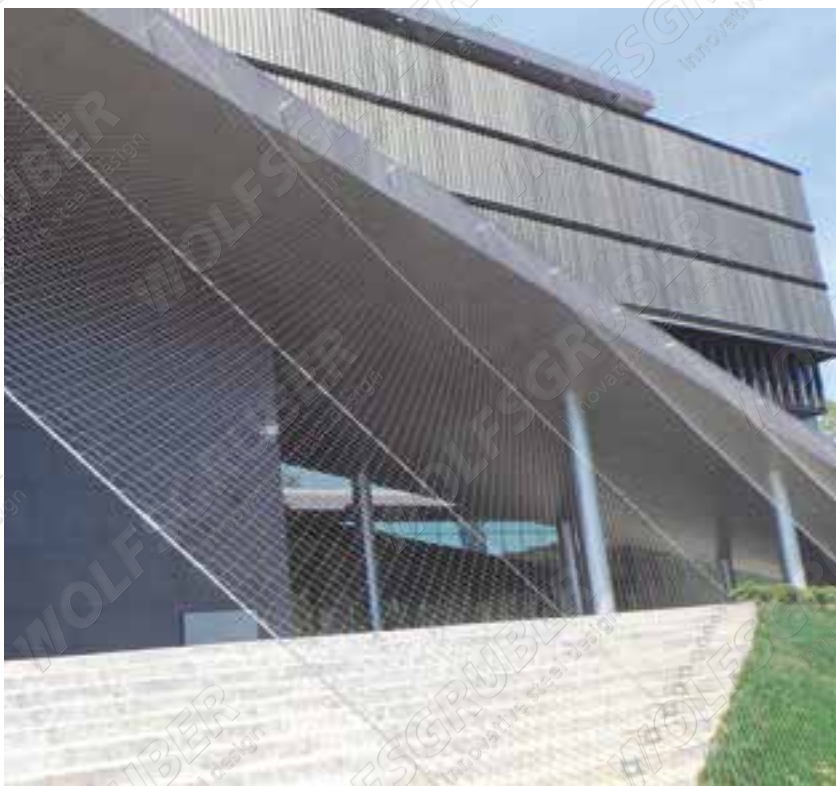
X-TEND CXE / I-SYS 800 m 2 , \diamond 80 mm, \circ 2 mm / \circ 6 mm
