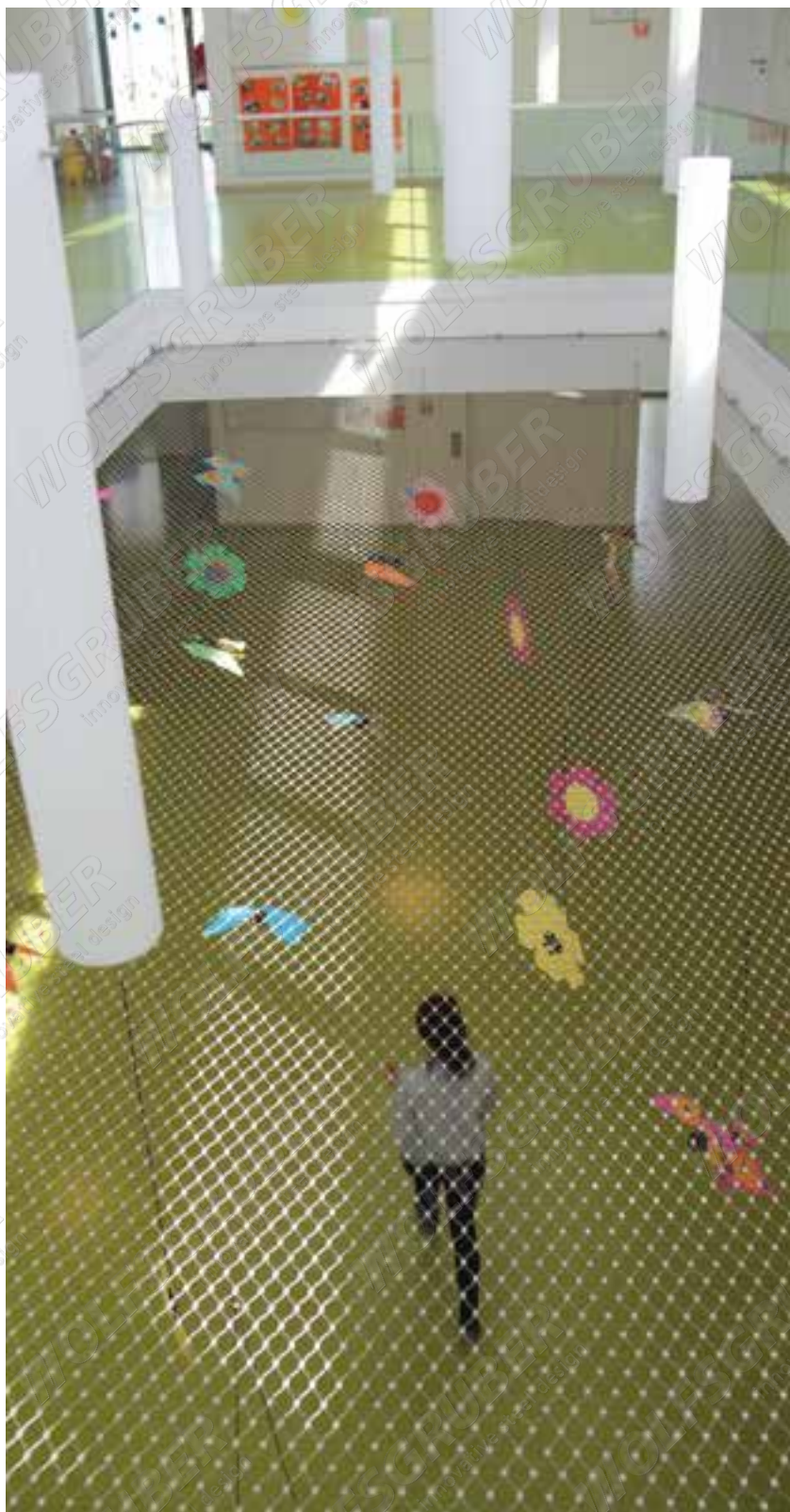
X-TEND CX / I-SYS 60 m 2 , \diamond 40 mm, \circ 2 mm / \circ 8 mm
