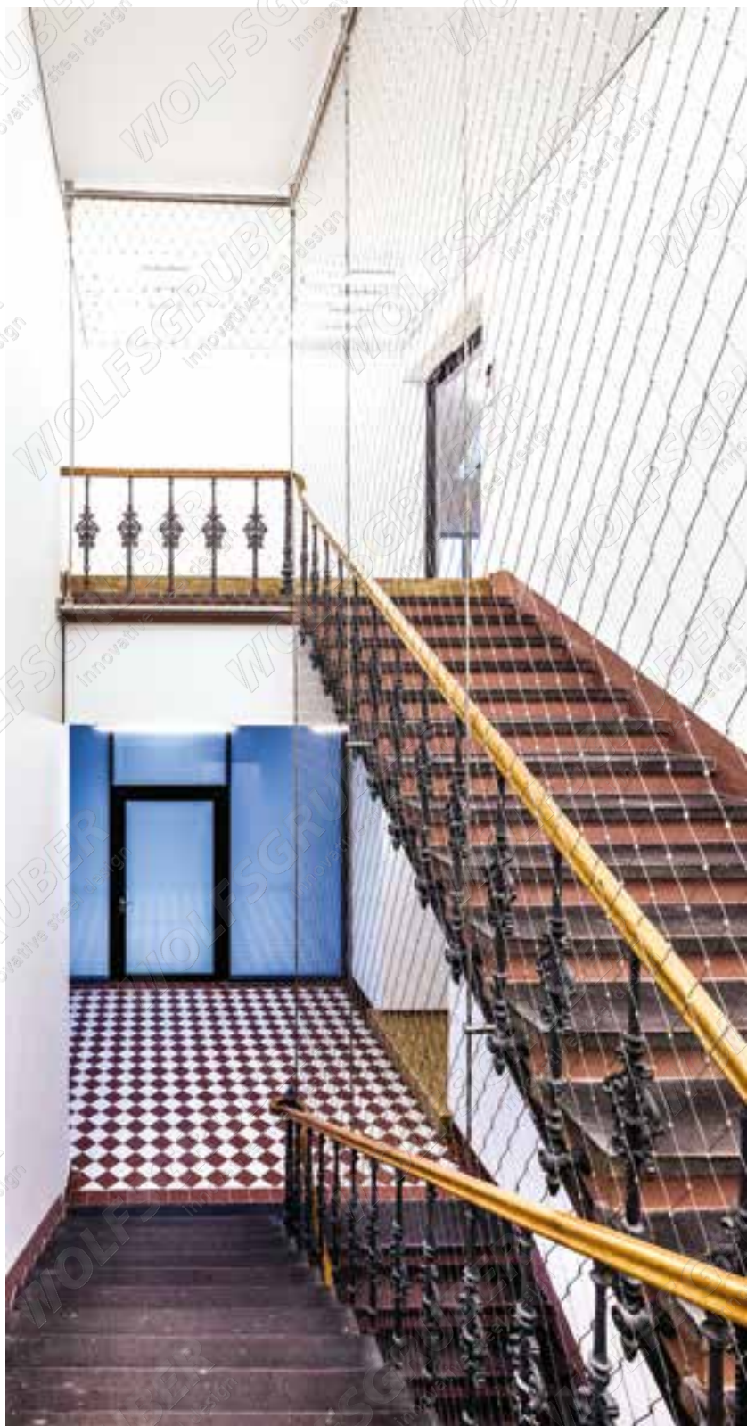
X-TEND CX / I-SYS 150 m 2 , \diamond 60 mm, \sigma 2 mm / \sigma 8 mm
